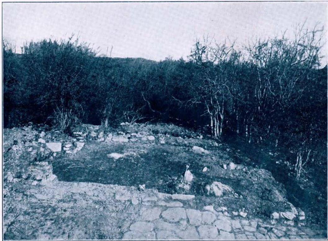
VIEW OF THE HOUSE "A" FROM THE SOUTH
