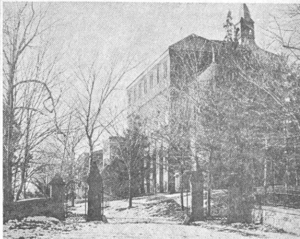
Elmhurst building, as seen through main entrance, may yield to student parking lots. —COWL photo by FRED LUMB
