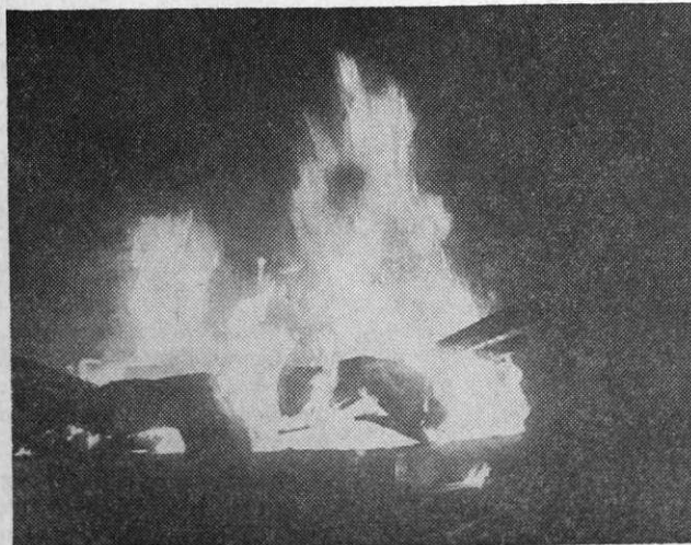
SUNDAY AFTERNOON FIRE at the library construction site.
