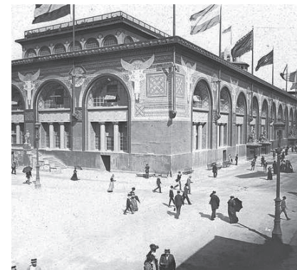
Figure 8: Detail of the Transportation Building, Chicago, Illinois, 1893, (Destroyed)
