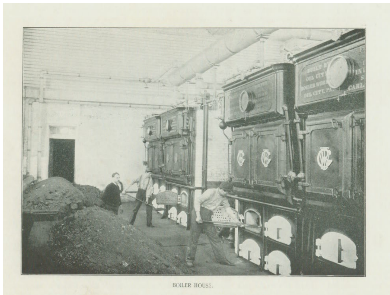
Image 8: Students at work in the Boiler Room
