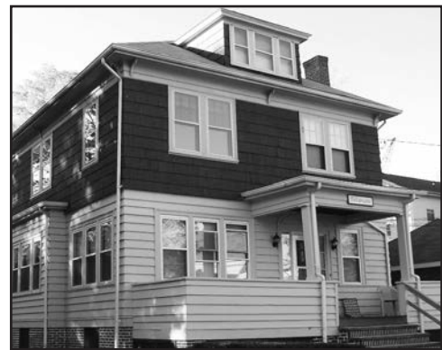
TOLLAMORE 138-140 Radcliffe Avenue
