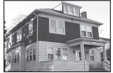
TOLLAMORE 138-140 Radcliffe Avenue
