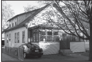
KILLARNEY 93 Pinehurst Avenue
