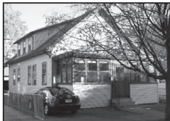
KILLARNEY 93 Pinehurst Avenue
