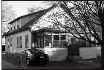
KILLARNEY 93 Pinehurst Avenue
