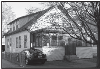
KILLARNEY 93 Pinehurst Avenue
