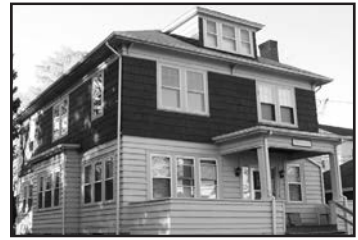
TOLLAMORE 138-140 Radcliffe Avenue
