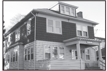
TOLLAMORE 138-140 Radcliffe Avenue
