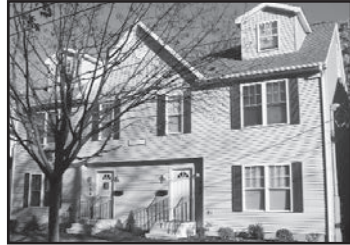
CASTLEBAR 127-129 Pinhurst Avenue
