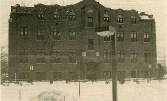
Stephens Hall is one of the numerous buildings containing asbestos on the PC campus which is targeted for asbestos abatement activities. (Photo by Mary Ann Doyle).
