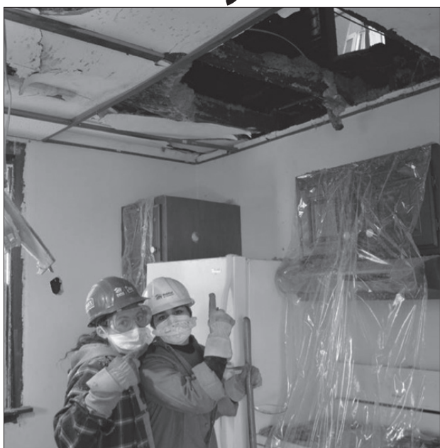
Megan Yaeger '19 and Annie Butler '19 pose during demolition.
